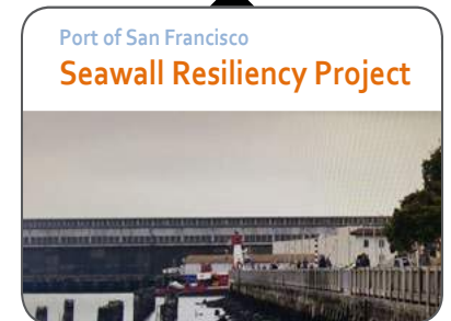
2017 Seawall Resiliency Project, SF Port
