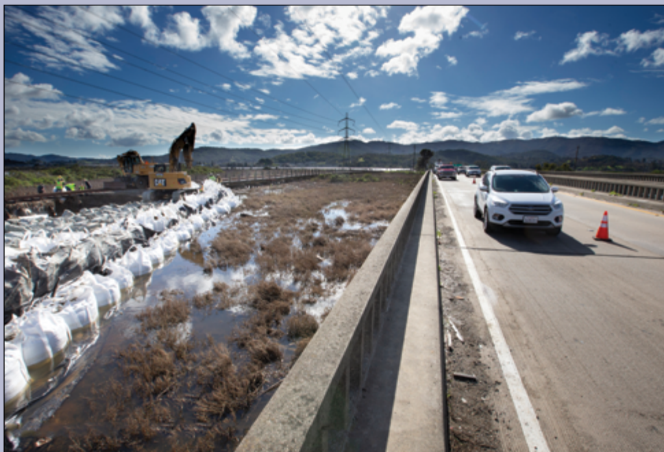
Levee repair after recent flooding on Highway 37. Photo: Caltrans/John Huseby
