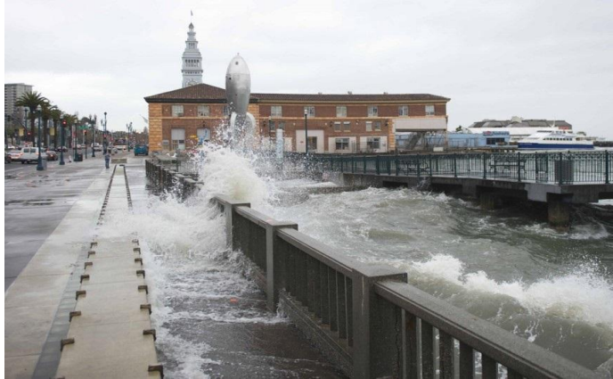
Photo: Port of San Francisco
